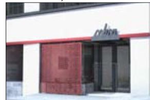
CCHCA San Francisco, CA Exterior Security Gates
