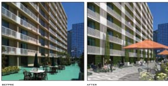
Holiday Inn Renovation Study San Francisco, CA Exterior Balcony Rails
