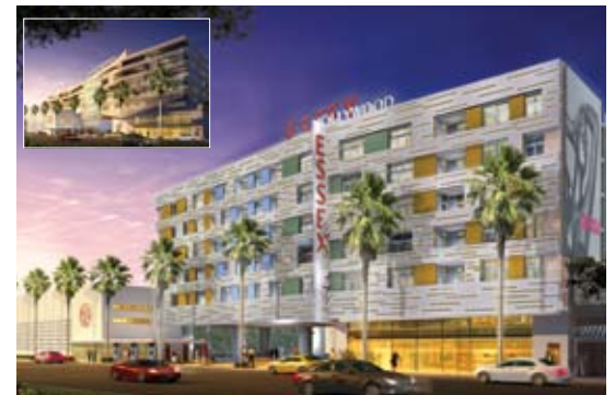
Essex Apartments Hollywood, CA Exterior Wall Screens
